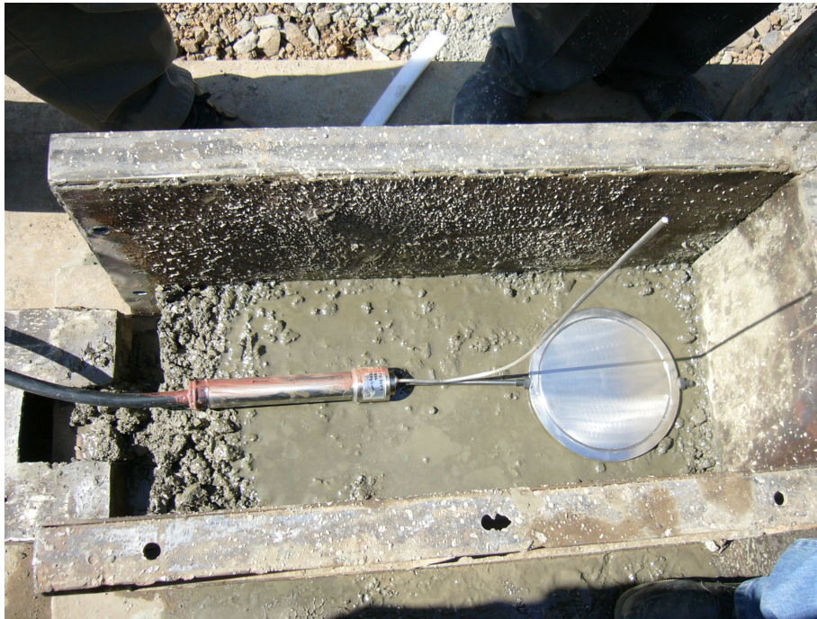
Fig11: Installation of stress meters in a concrete block to be later shifted to its location in RCC dam
