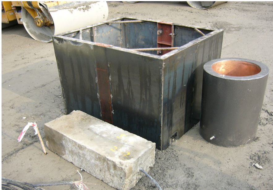
Fig 12: Formwork for installation of strain meter group at RCC dam site. The stress meter cast in a concrete block and the no-stress-strain container can also be seen.
