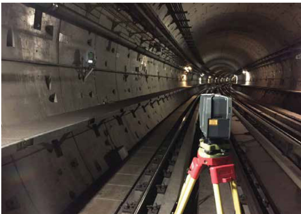
Fig. 12. Laser scanner for tunnel deformation monitoring
