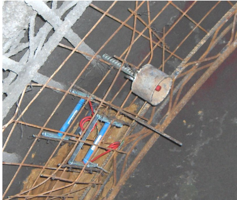
Fig. 1. A pair of shotcrete strain gages and convergence bolt of an optical target installed before shotcreting of an NATM tunnel
