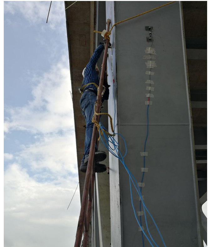
Installation of strain gage at diagonal girder
