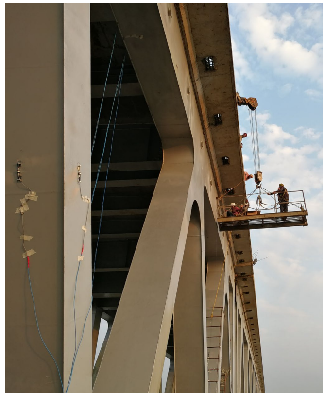
Installation of thermocouple at top cross girder
