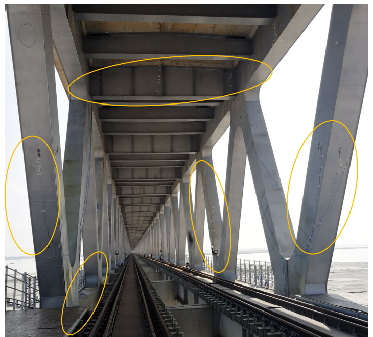
Strain gages and thermocouple installed on bridge
