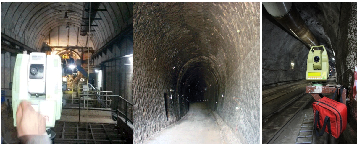
Automatic total station for tunnel 3D deformation monitoring
