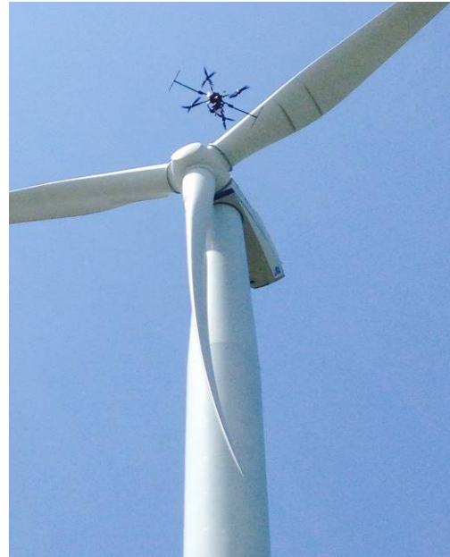
Wind turbine inspection using drone
