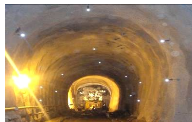
Prism target in HRT at Dagachhu HEP, Bhutan
