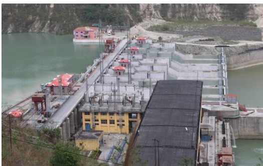
Teesta concrete gravity dam, India
