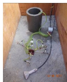
Strain gage rosette and piezometer being installed at Nam Pha dam, Laos
