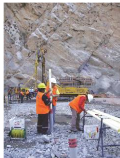
Inclinometer being installed in EL Platanal rockfill dam, Peru
