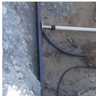
Soil extensometer being installed in a earth and rockfill
