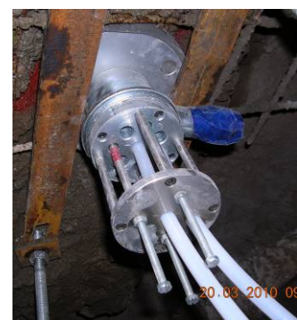
BHE and load cell in powerhouse at Koprubasi HEP, Turkey
