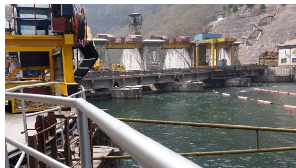
Chukha concrete gravity dam, Bhutan
