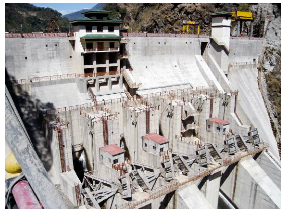
Tala concrete gravity dam, Bhutan
