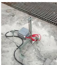
Triaxial jointmeter installed at Teesta III
