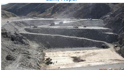
Work in progress at Salma Dam, Afghanistan
