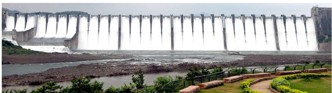
Sardar Sarovar concrete gravity dam,
