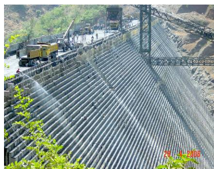
Ghatgar RCC dam, India
